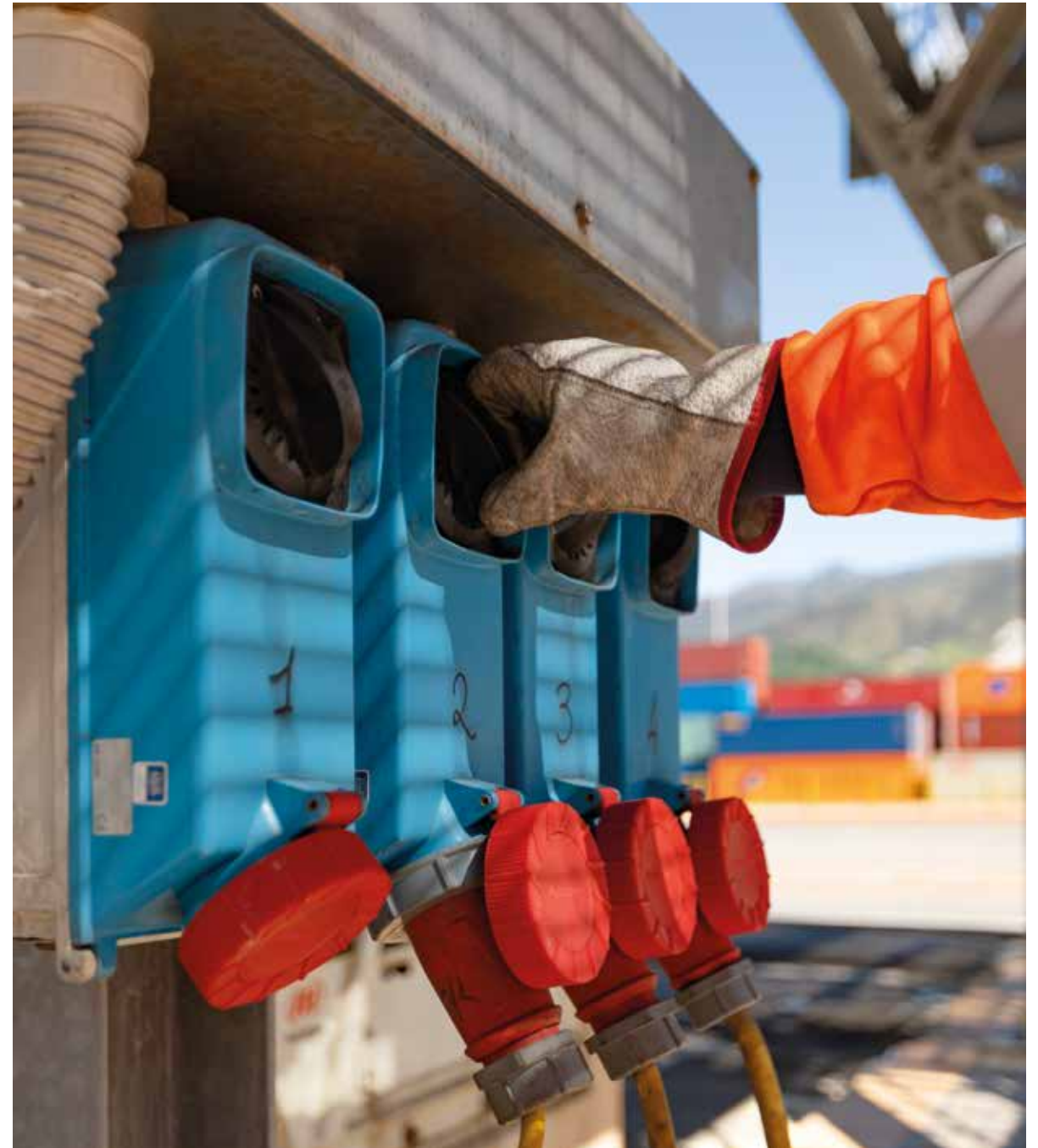
PSA Genova Pra': an operator at work in the reefer yard area, powered by electricity..
